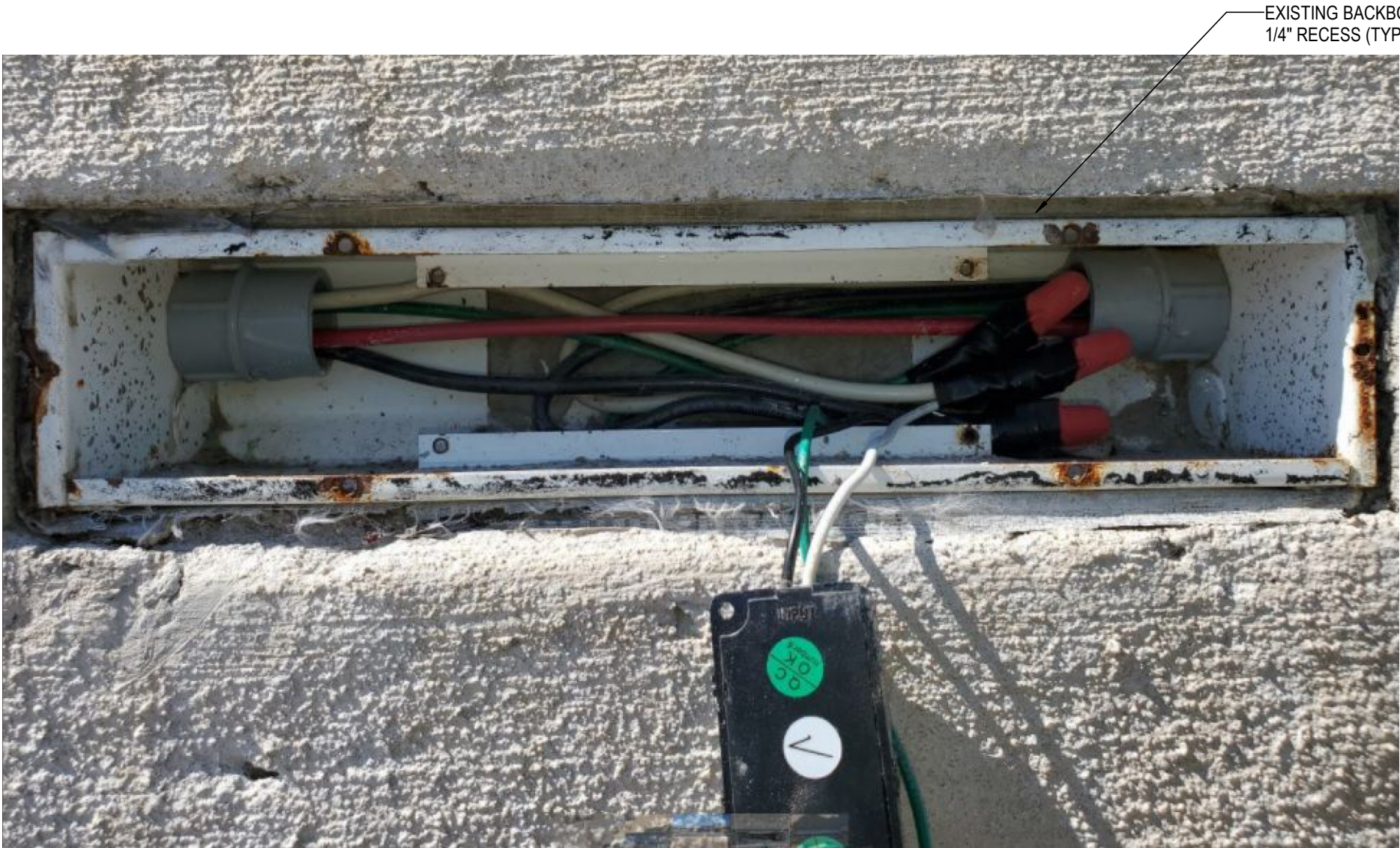
EXISTING CONDITIONS - BACKBOX NOT TO SCALE
